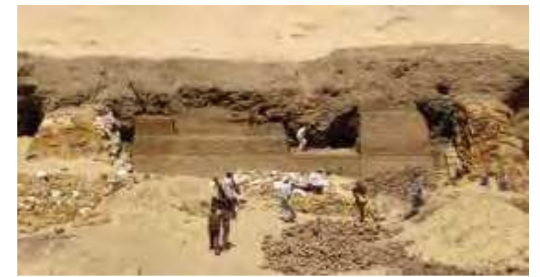
Fig.4 East enclosure wall showing the process of constructing the mud-brick foundation system (credits: Anthony Crosby, 2010)
