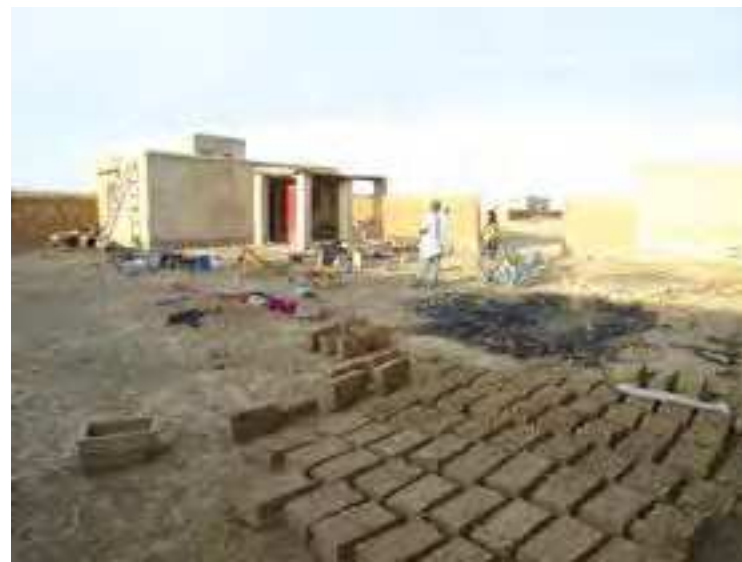
Fig.6 Adobes ready for the recovery (credits: CRAterre, Thierry Joffroy, 2011)
