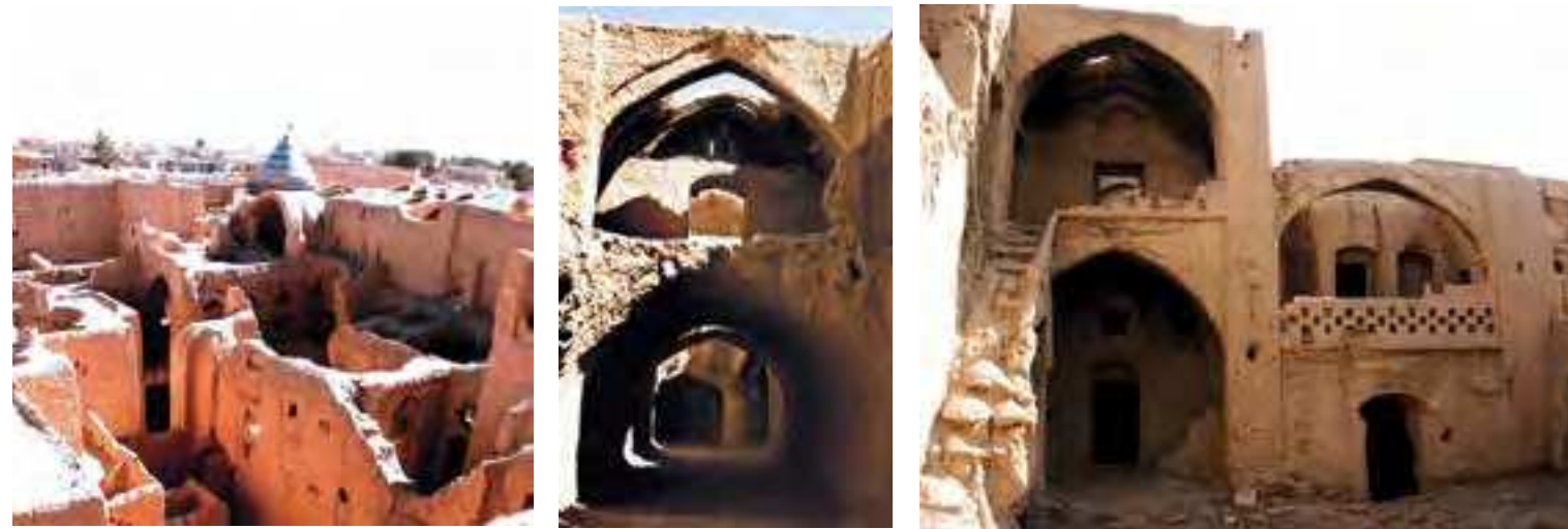
Fig.2, Fig.3 and Fig.4 Historical structures in Moorcheh Khort, Iran (credits: M. R. Manouchehri, 2008)
