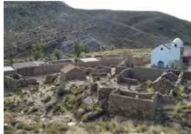
Fig.4 Hamlet and small church in La Cueva, Argentina, constructed of adobe, stone and clay, earthen plasters, and terracotta tiles roof (credits: Rodolfo Rotondaro, 2009)
