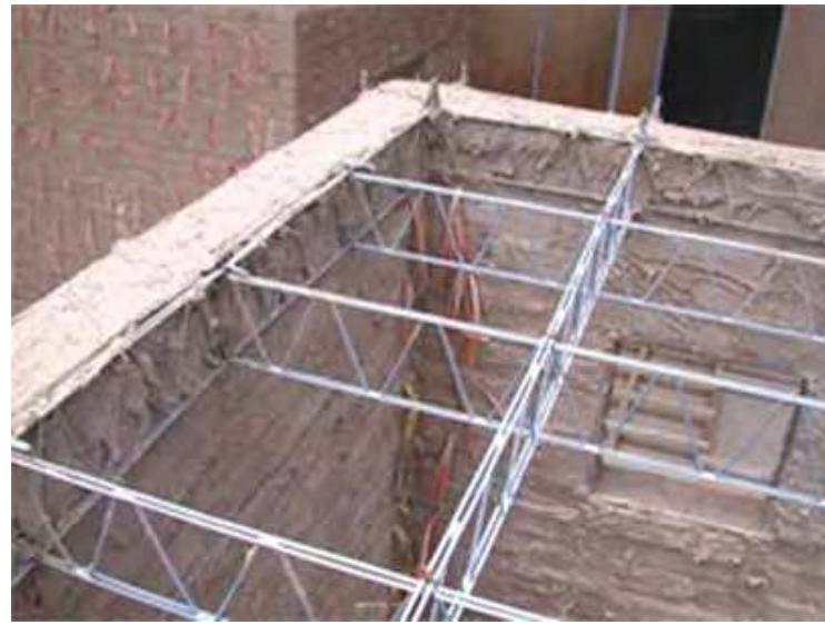
Fig.3 The unreinforced corner had no major complications. Note that the rack truss, which functions as the ceiling joists, also functions as a perimeter beam (credits: Adell, 2008)
