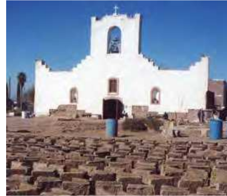
Fig.2 Nuestra Señora de la Limpia Concepción de Lós Piros de Socorro del Sur in Socorro Texas, surrounded by adobe bricks handmade by the community and other volunteers (credits: Pat Taylor, 1994)
