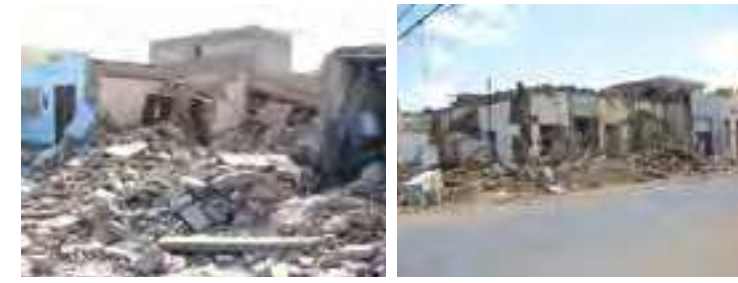
Fig.1 Collapsed houses during the earthquakes of Pisco, Peru, 2007 and Maule, Chile, 2010 (credits: J. Vargas-Neumann, 2007 y 2010)
