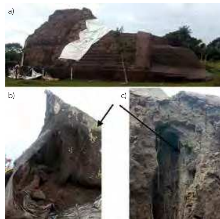
Fig.6 La Joya Pyramid in September 2010, after hurricane Karl: a. west façade with torn tarpaulins, southern sector (on the right) with polymer layer in good condition, b. collapse of north profile fill, arrows indicating weeds and roots, c. detail of weed roots in old crevices, originally filled with sand (credits: Annick Daneels, from project authorized by the Archaeology Council of Mexico's National Institute of Anthropology and History)
