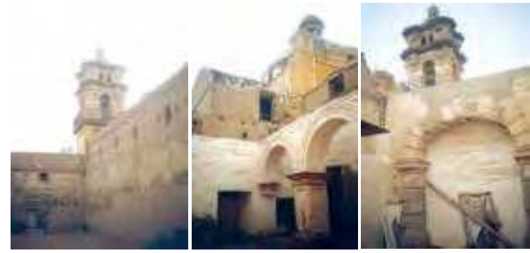
Fig.3 The Compañía Church, Pisco: a) Adobe walls coated with cement at the bottom; b) Earthen-framework vault and dome left weathering without an earthen coating; c) Adobe arch with cementitious-coating renovation (credits: Pedro Hurtado Valdez, 2007)
