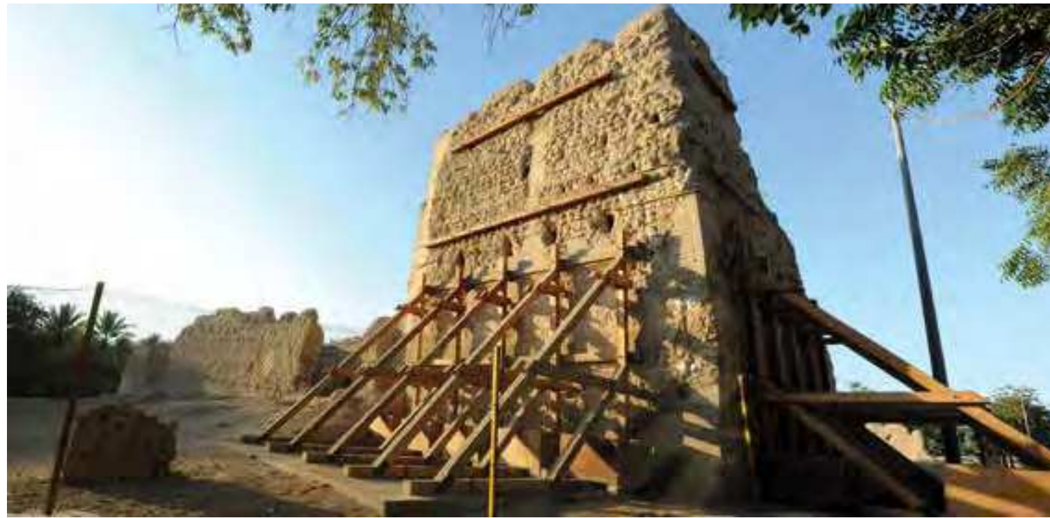
Fig.4 Abdullah Bin Salem Al-Darmaki House showing steel pinning and shoring (credits: Salman Muhammad © ADACH, 2011)
