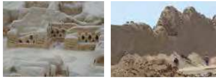
Fig.8 A sacrifice layer of gravel is used to protect the top of the walls. Audiences sector, Tschudi palace (credits: Mariana Correia, 2005) Fig.9 Reconstruction of the surrounding wall in Velarde palace, Chan Chan (credits: Luis Guerrero, 2007)
