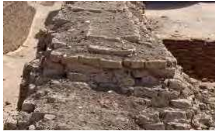
Fig.6 Comparison of mud-brick protective cap and existing wall top (credits: Anthony Crosby, 2005)
