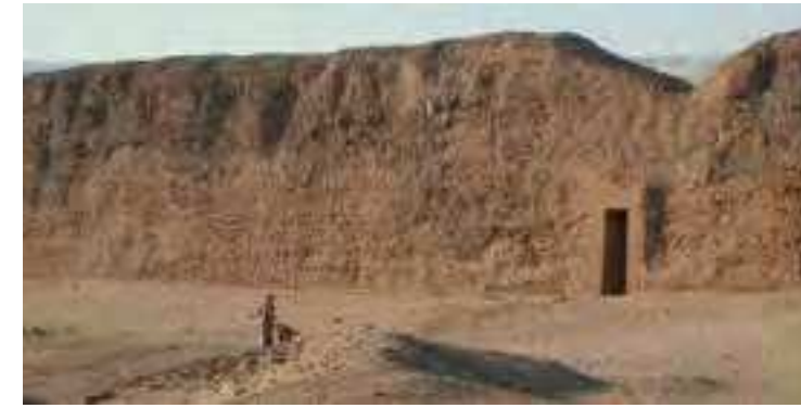
Fig.7 The west enclosure wall from the north after completion of the west gateway stabilization and restoration (credits: Anthony Crosby, 2010)
