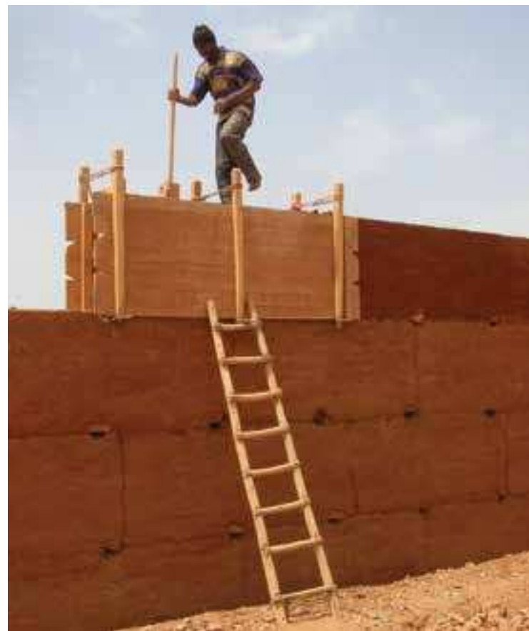
Fig.4 Rammed-earth masonry construction in the Drâa Valley (credits: Saverio Mecca, 2007)
