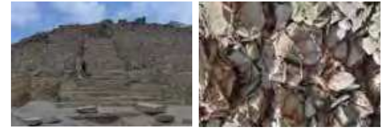
Fig.1 Staggered Pyramid "La Galería", in Caral, from 3,000 BC. The complex is built in stone masonry, earth mortar and wattle-and-daub (credits: Julio Vargas, 2011)
