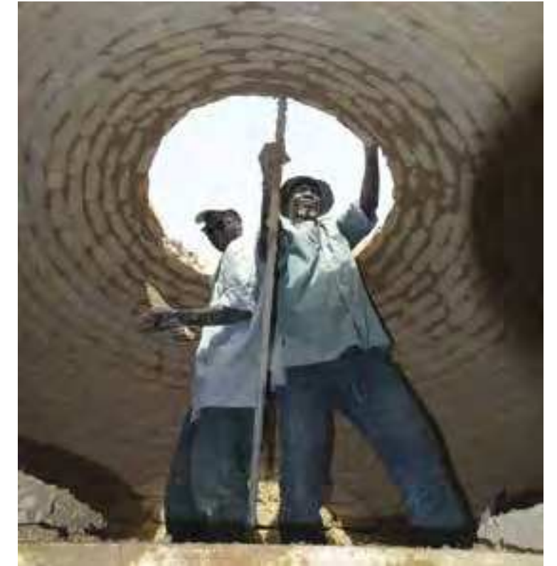
Fig.5 Construction of cupolas (credits: CRAterre, Laure Cornet, 2010)
