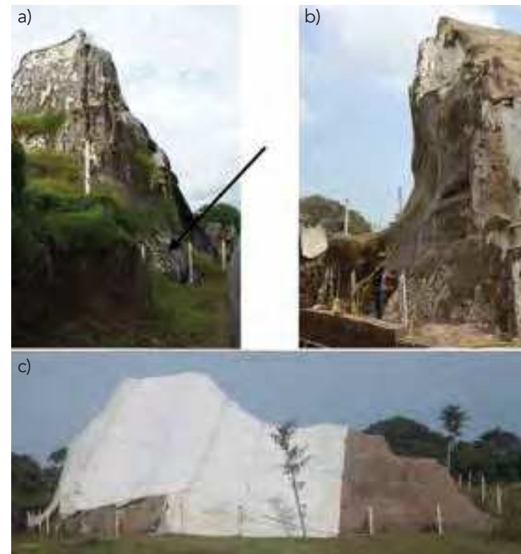
Fig.4 La Joya Pyramid in spring 2010: a. arrow indicates collapse of north retaining wall due to weeds, b. geotextile applied directly to north profile, c. west façade protected by tarpaulins, whereas for the southern sector (on the right) with the new sacrificial layer with vinyl polymer (credits: Annick Daneels, from project authorized by the Archaeology Council of Mexico's National Institute of Anthropology and History)
