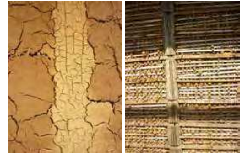
a) Shrinkage fissures resulting from drying of the first earthen layer; Fig.4a) b) Appearance of the inboard side (credits: Akemi Hijioka, 2010) Fig.4b)
