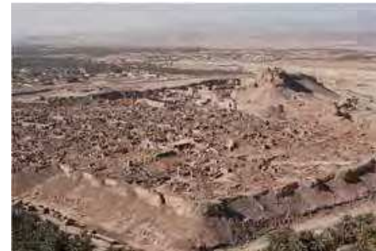
Fig.1 The Bam citadel in 2004 after the 2003 earthquake (credits: RPBCH, 2011)
