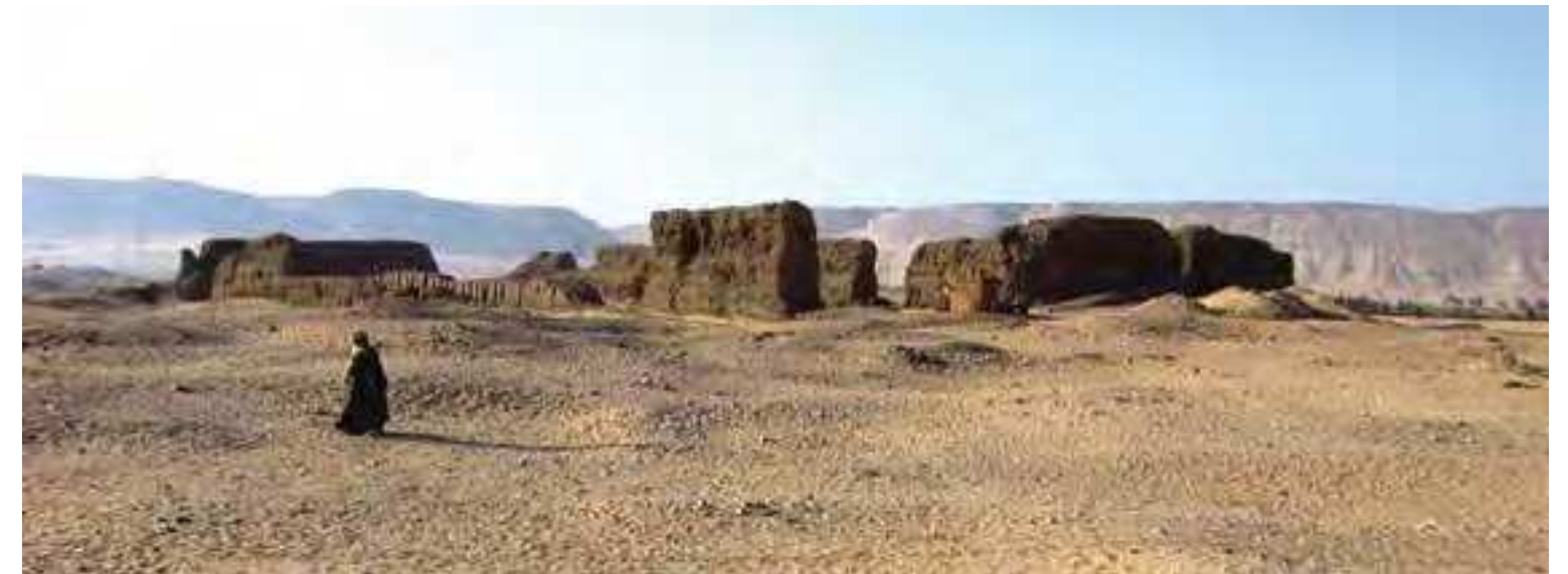
Fig.1 Shunet el Zabib, the funerary enclosure of Khasekhemwy from the north, with mud brick walls 11 meter high (credits: Anthony Crosby, 2001)
