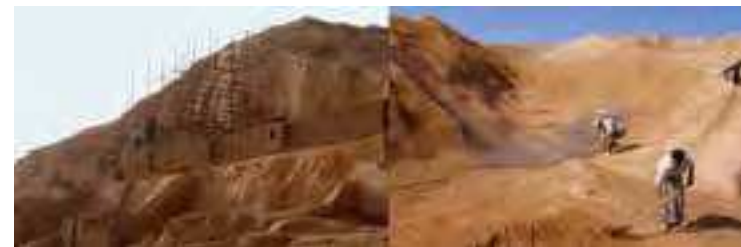
Fig.2 Surface protection and visual reintegration of the peak of Tchogha Zanbil Ziggurat by Kahgel (credits: The World Heritage of Tchogha Zanbil, 2004)
