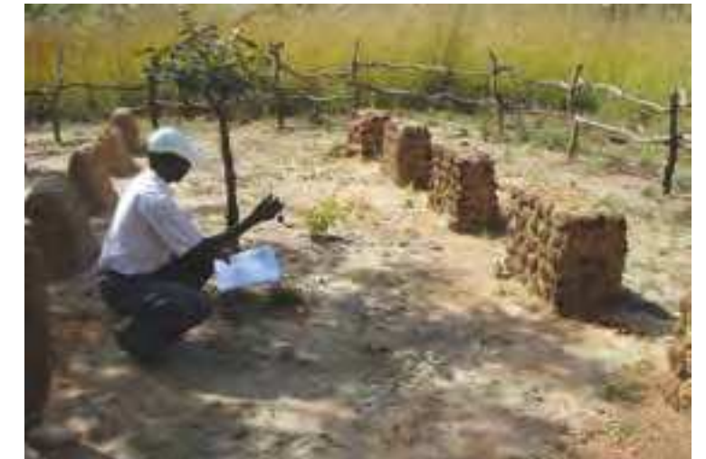
Fig.6 Preventive measure with sacrificial capping, Fayaz Tepa, UNESCO-Japan-Fund-in-Trust project, Uzbekistan (credits: Thierry Joffroy, 2003)
