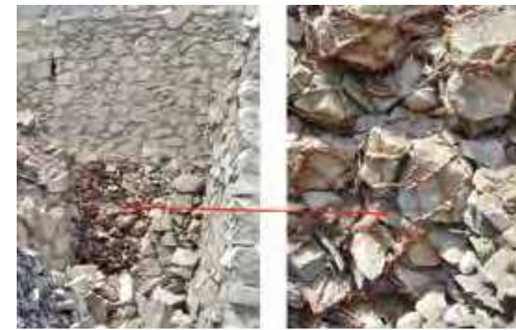
Fig.2 Reed shicras providing stability to the fill. There are fills with balanced vertical flat edges, which supported the upper overburden and the expansion of the shicras' area (credits: J. Vargas-Neumann)
