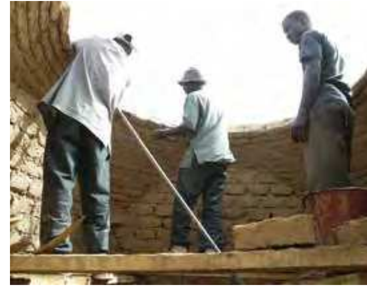
Fig.4 Construction of cupolas (credits: CRAterre, Laure Cornet, 2010)
