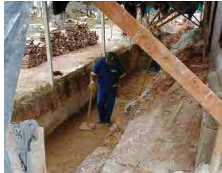
Fig.2 Rammed-earth veneer to protect the foundations of the Igreja Matriz De Santo Antonio (credits: Silvia Puccioni, 2000)
