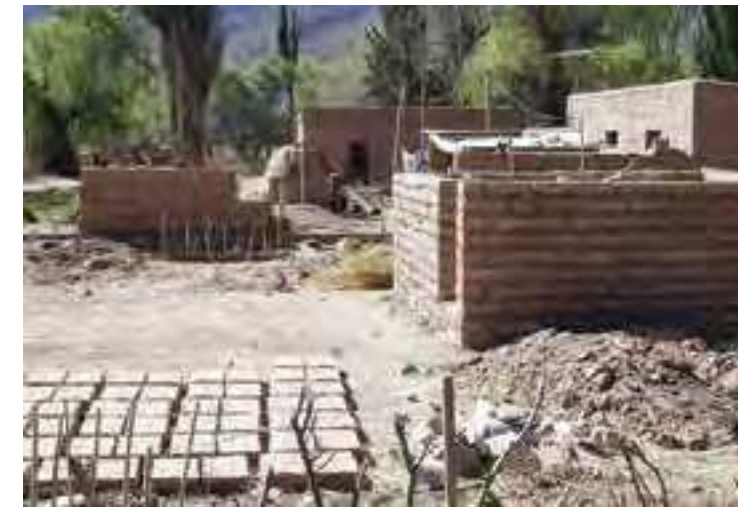
Fig.1 Self-construction of a domestic housing using adobe, and terracotta tiles on hollow reed in El Perchel, Argentina (credits: Rodolfo Rotondaro, 2009)
