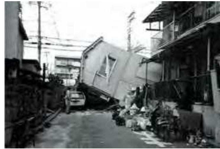
Fig.3 Kobe 15th Mansion (protected heritage) destroyed by Kobe Earthquake, M.7.3, January 17, 1995 caused liquefaction of the ground (credits: K.Masuda 1995)
