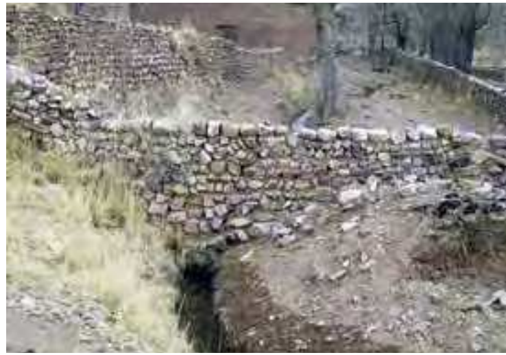
Fig.3 House fence of stone and clay over an irrigation ditch outside Iturbe, Argentina (credits: Rofolfo Rotondaro, 2009)
