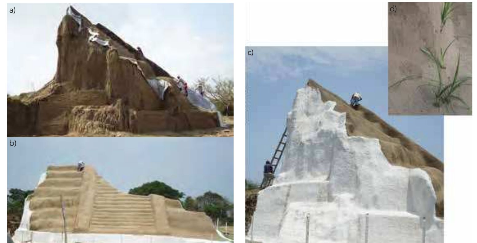
Fig.5 La Joya Pyramid in spring 2009: first preservation experiment: a) retaining walls at the foot of west façade and on the north profile, placing of geotextile and protective layer; b) west façade after preservation; c) north profile after preservation and d) weeds growing through geotextile and sacrificial layer (credits: Annick Daneels, from project authorized by the Archaeology Council of Mexico's National Institute of Anthropology and History)
