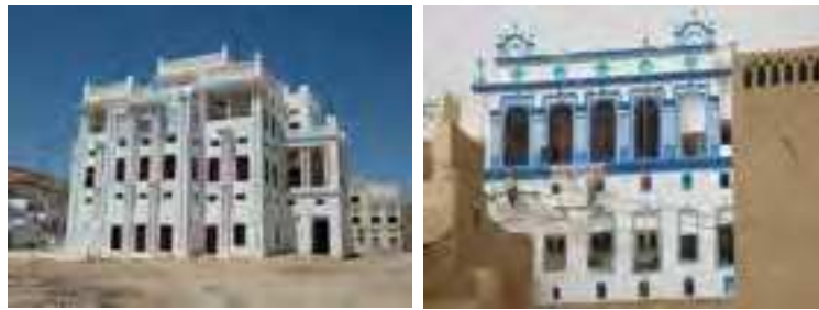
Fig.2 Al-Riyadh following restoration of the exterior (credits: Pamela Jerome, 2010)
