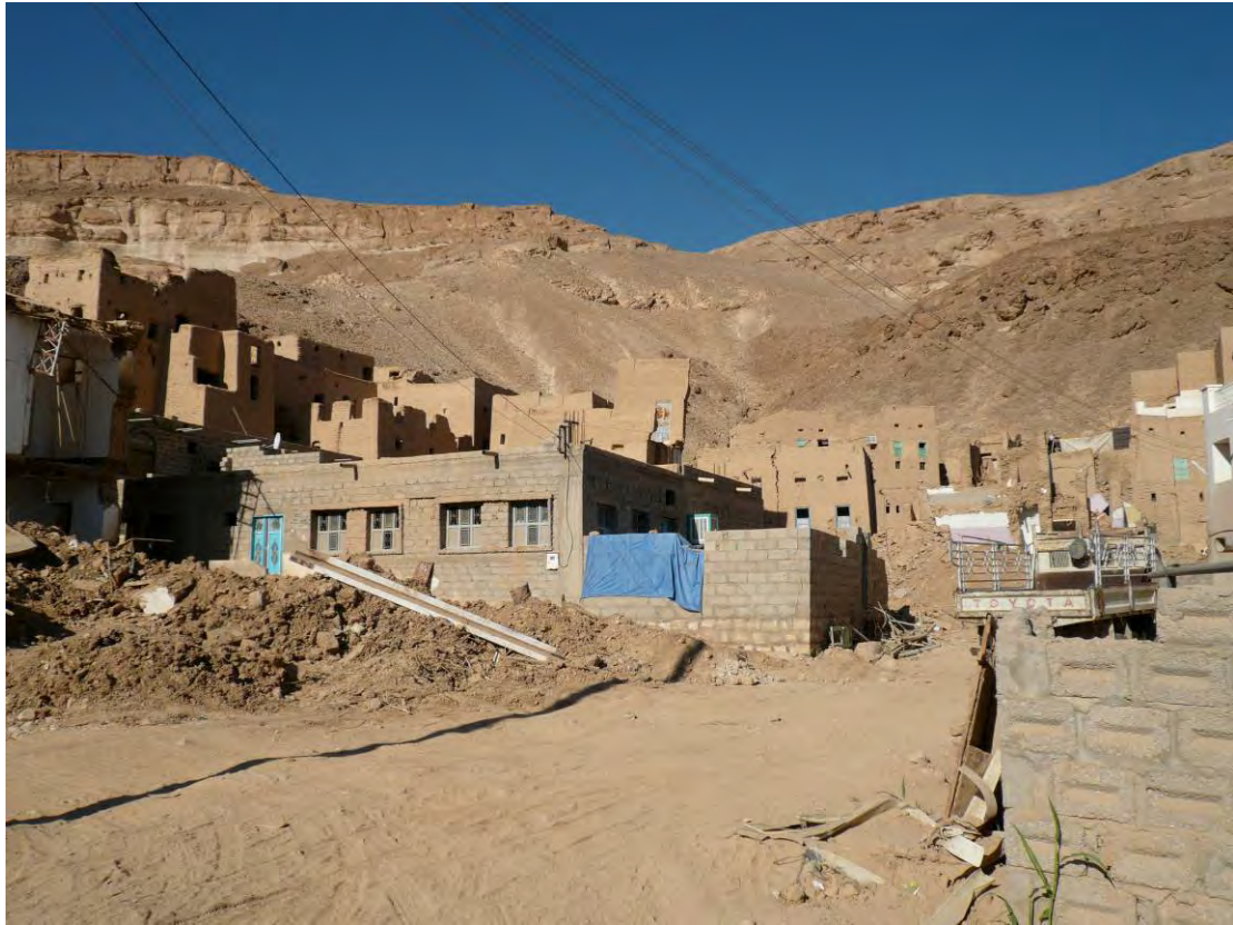
Fig. 4 – Recent incursions of concrete construction into traditional villages caused damage to surrounding mudbrick structures during the flood through turbulence and rebound effect. This example is in al-Jihad to the east of Tarim. (credits: Pamela Jerome, 2008)
