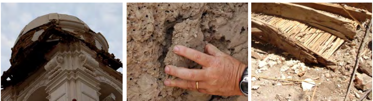
Figure 6, left: Upper dome of Hacienda San Jose Chapel where connections deteriorated inducing loss of structural integrity. (Credits: J. Paul Getty Trust, 2007)
