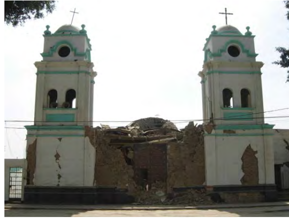
Figure 5: Church of Guadalupe after the Pisco earthquake where out of plane of collapse of front facade induced partial collapse of the quincha vault. (Credits: J. Paul Getty Trust, 2007)
