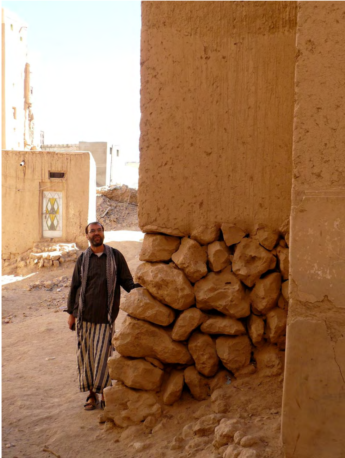
Fig. 3 – Dry rubble-stone foundations in the Wadi Do'an can be over 1.50 m in height, and in this case, closer to 1.80 m. Pictured here is a tower house in the notable village of Budha located in the right branch of the Wadi Do'an. (credits: Pamela Jerome, 2008)
