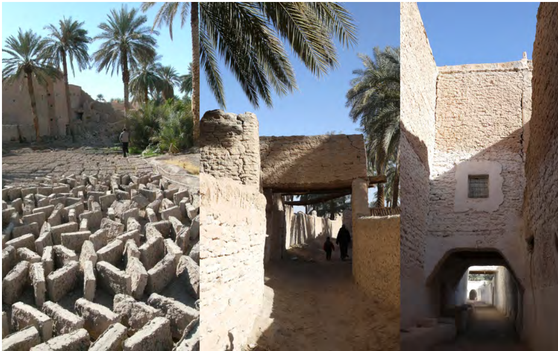
fig.2 : Optimization of local resources : adobe production in the palm-grove to progressively build a high density urban pattern. (credits : Thierry Joffroy, CRAterre, 2008)
