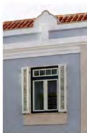
Fig.2 - Pormenor Fachada Principal
