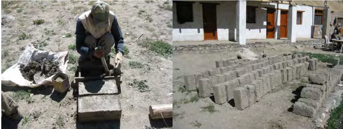
Fig.4 - Studying the vernacular building technologies: production of the the pakbu , the local mud brick (credits: Désirée De Antoni)
