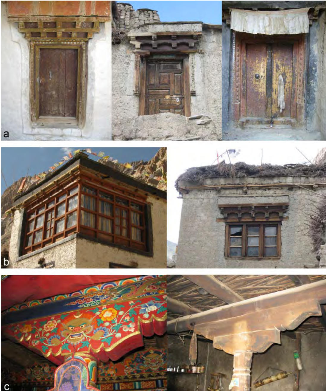
Fig.5 - Understanding the architectural details: (a) doors, (b) windows, (c) capitals (credits: Giulia Bravo, Désirée De Antoni)
