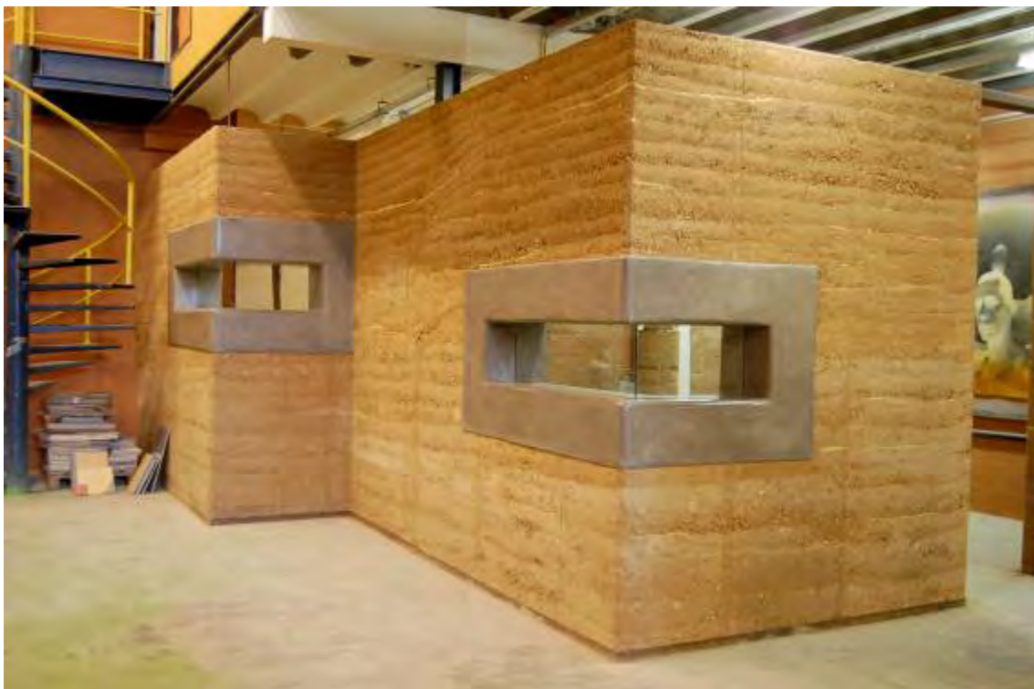
Fig. 6 – Office Amsterdam, the Netherlands (credits: Leemwerk).
