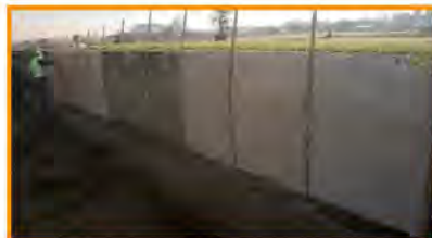
Figure 5 – Render panels over adobe wall
