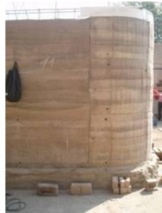
(Fig. 3) Junta constructiva vertical
