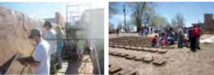
Fig.3 Volunteers plastering walls at San Miguel Chapel in Santa Fe, NM (credits: Jake Barrow, 2011) Fig.4 Volunteer day making adobes at Old Trading Post at Santo Domingo Pueblo (credits: Jake Barrow, 2011)
