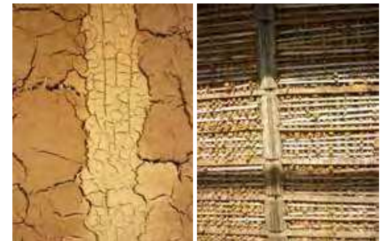
a) Fig.4a) Shrinkage fissures resulting from drying of the first earthen layer; Fig.4b) Appearance of the inboard side (credits: Akemi Hijioka, 2010)
