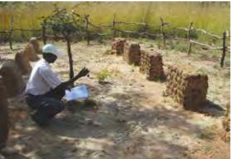
Fig.6 Preventive measure with sacrificial capping, Fayaz Tepa, UNESCO-Japan-Fund-in-Trust project, Uzbekistan (credits: Thierry Joffroy, 2003)
