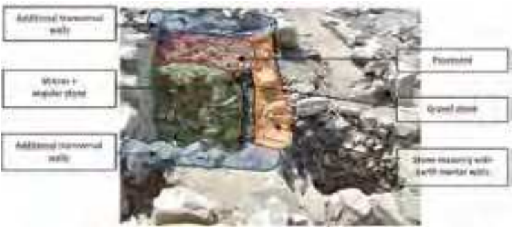
Fig.4 Alternative to the first type of nucleus structure (credits: J. Vargas-Neumann)
