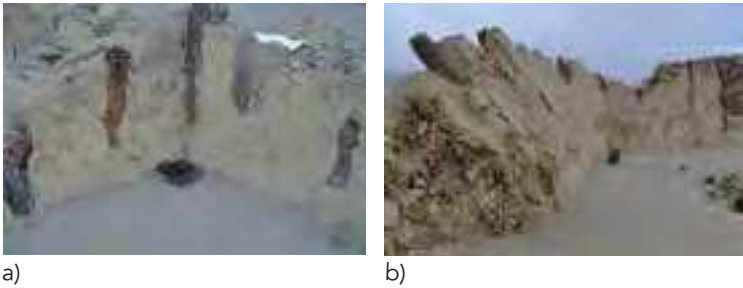
Fig.5 The oldest example of quincha found in America. a) Quincha structures; b) Trusses (credits: J. Vargas-Neumann)
