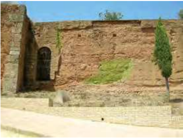
Fig.3 Damage in earthen the fabric of the wall between Towers 6 and 7 in 2009 (credits: A. González, 2009)
