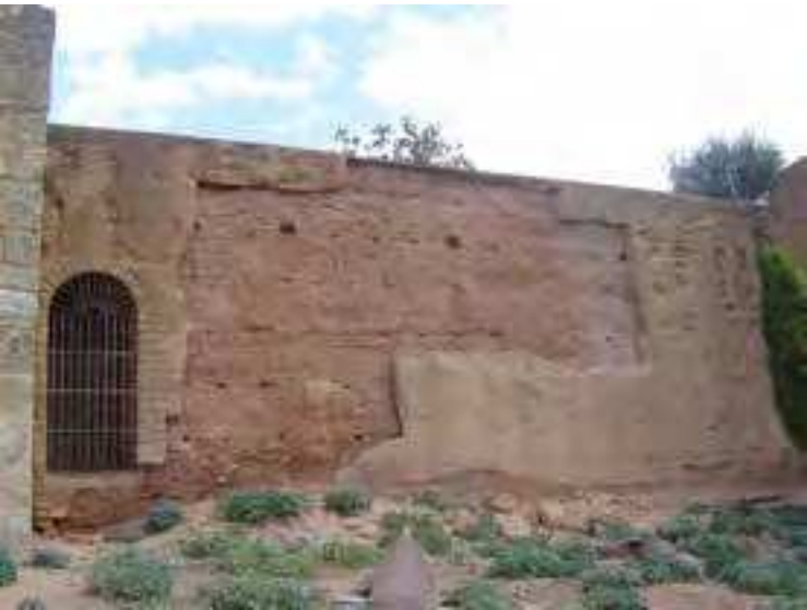
Fig.3 Damage in earthen the fabric of the wall between Towers 6 and 7 in 2009 (credits: A. González, 2009)
