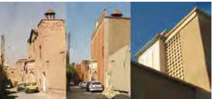
Fig.1 Experience of surface protection in Isfahan, a) and b) French School, Jolfa, before (2002) and after the repair of Simgel decorations (2011); c) application of tile and brickwork in combination with gypsum plasters and mud coatings in the façade of a house in the neighborhood of Meidan Emam (credits: Reza Vahidzadeh, 2011)
