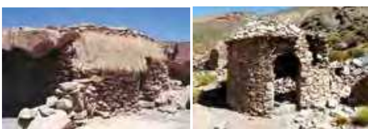
Fig.2 One puesto built with pirca seca (credits: Jorge Tomasí) Fig.3 A case of a circular kitchen in a rural house, with a false vault in stone (credits: Jorge Tomasí)
