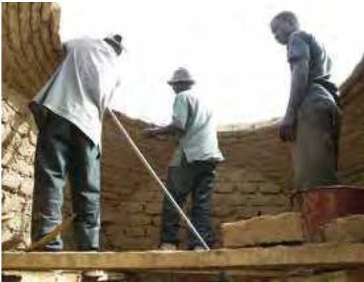
Fig.4 Construction of cupolas (credits: CRAterre, Laure Cornet, 2010)
