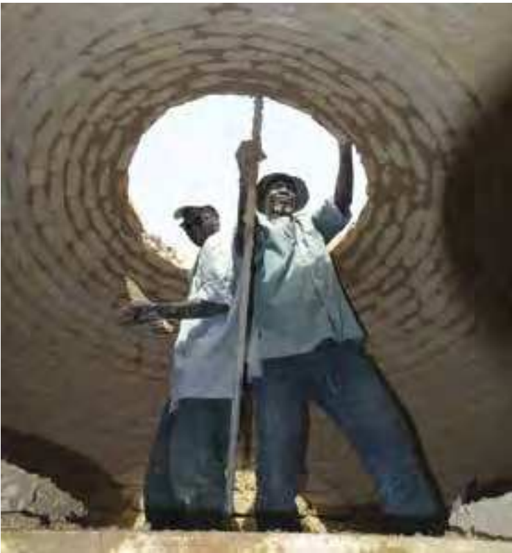
Fig.5 Construction of cupolas (credits: CRAterre, Laure Cornet, 2010)
