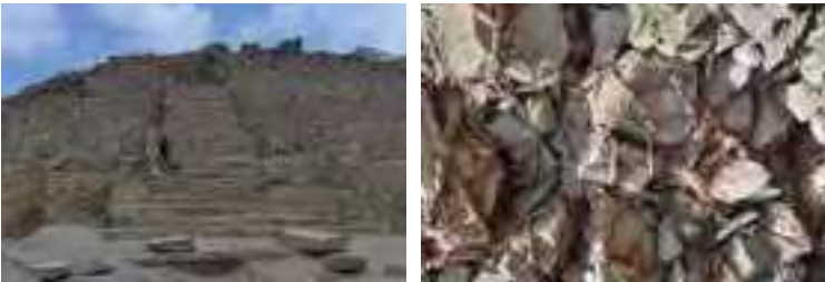
Fig.1 Staggered Pyramid “La Galería”, in Caral, from 3,000 BC. The complex is built in stone masonry, earth mortar and wattle-and-daub (credits: Julio Vargas, 2011)
