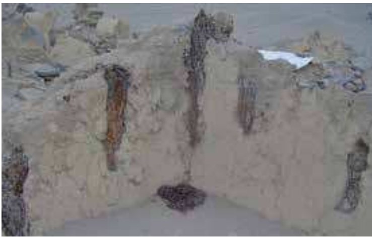
Fig.3 Remnants of shicras used for bagging stones for stable pyramid cores (credits: Julio Vargas, 2011) Fig.4 Quincha (wattle-and-daub) is an earthquake-resistant composite technology (credits: Julio Vargas, 2011)
