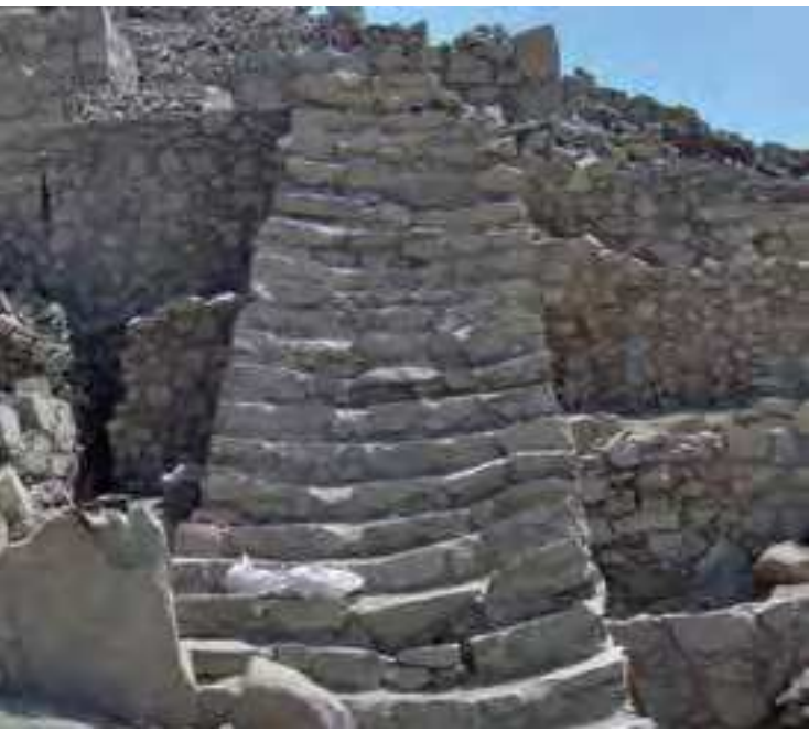
Fig.5 Unstable stairs requiring the renewal of shicras (credits: Julio Vargas, 2011)
