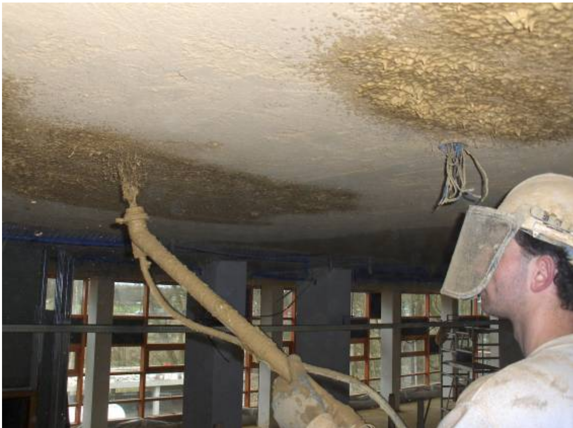
Fig. 2 – Spraying earthplaster WWF Zeist, the Netherlands (credits: Michel Leeman).
