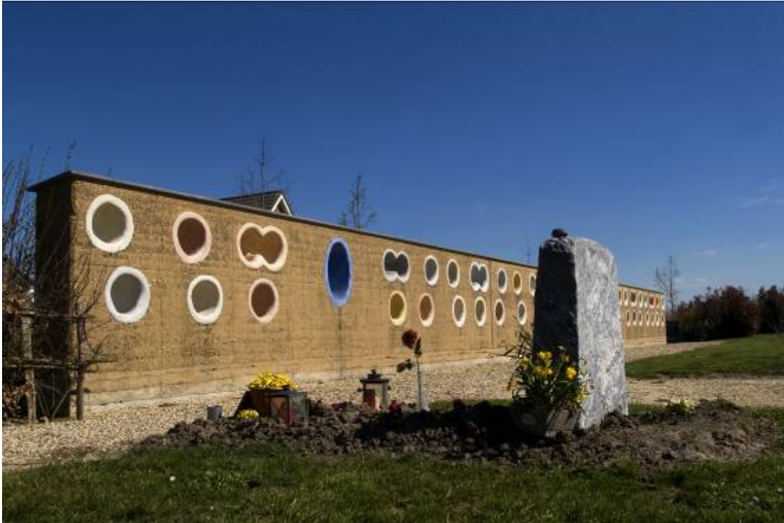
Fig. 4 – Rammed earth wall cemetery Spijk, the Netherlands (credits: Pieter Boer).
