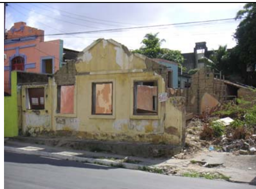
Fig.2 This 19 th century wattle and daub family home came down after thieves took its roof. It stood many years of neglect due to family estate litigations. This fine example of earth architecture has now been totally lost after the 2009 rains that turned it into a pile of rubble. County of Casa Forte , Recife. (Credits: Plínio Santos-Filho, 2008)
