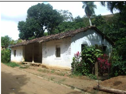
Fig.1 Wattle and daub 19 th century train station in the old district of Macacos (now called Guabiraba , Recife.) A lime plaster outer layer protects the external walls from the tropical rains. The building has been preserved by the constant use of the original station keeper's family and is now a residence. (Credits: Plínio Santos-Filho, 2007)
