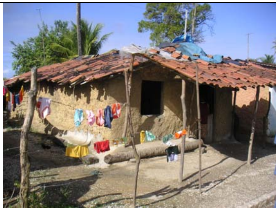
Fig.3 Typical wattle and daub house in the community of Povoação de São Lourenço. There is very little finish to either internal or external walls. Wood is extracted the mangrove sanctuary down hill, causing great environmental impact. The floor plan is a rather standard 5 m x 7 m outer shell, with one division for a bedroom and no bathroom. Usually there are no bathrooms, and when they do exist, they are external to the house and consist of an uncovered hole in the ground. Usually there is a very primitive wood stove, African style, behind the house. (Credits: Plínio Santos-Filho, 2009)
