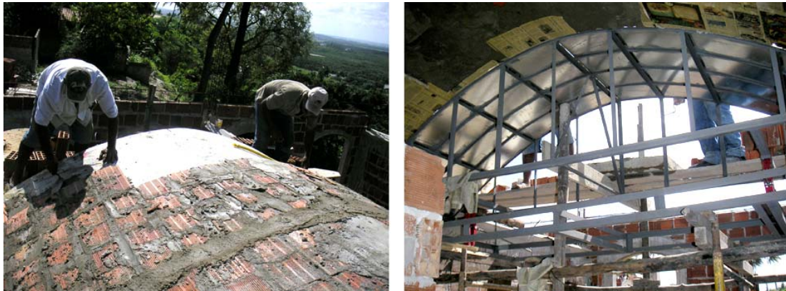
Fig.5. The 3.50 m roof span of the house is covered by an inverted gravitational catenary arch, and made out of standard 8 holes Brazilian fired bricks. (Credits: Plínio Santos-Filho, 2009)
