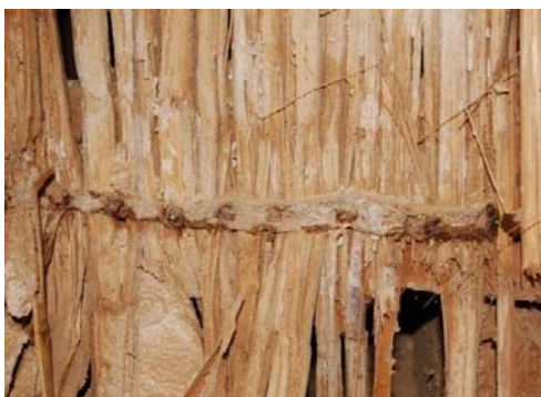
Figure 2: State of deterioration of Quincha panel at the Cathedral of Ica (Credits: INC Lima, 2007)
