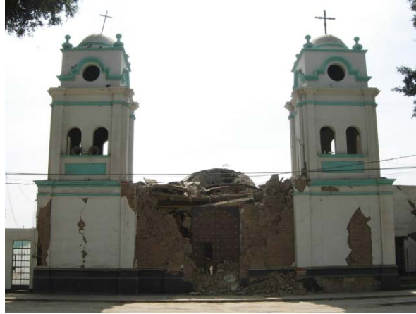
Figure 5: Church of Guadalupe after the Pisco earthquake where out of plane collapse of front facade induced partial collapse of the quincha vault. (Credits: J. Paul Getty Trust, 2007)
