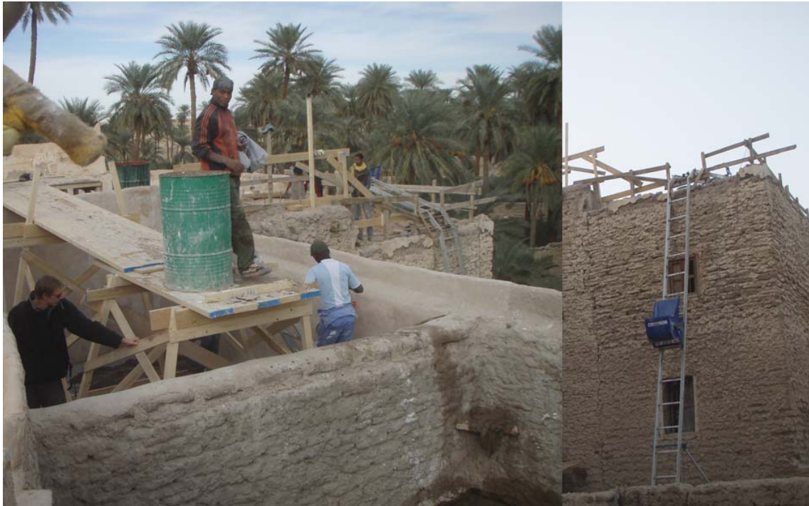
fig.4 : Mechanization and safety installations helped improve efficiency on Mazigh lodges' work-site (credits : Florian Herold, CRAterre, 2008)
