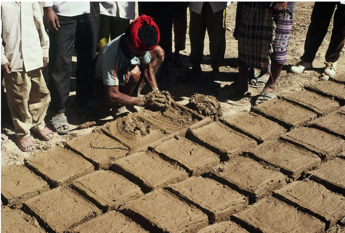
Fig. 6 – In Khoreibah, deep within Wadi Do'an, the mix for mudbricks is stiffer resulting in better quality. (credits: Pamela Jerome, 1997)
