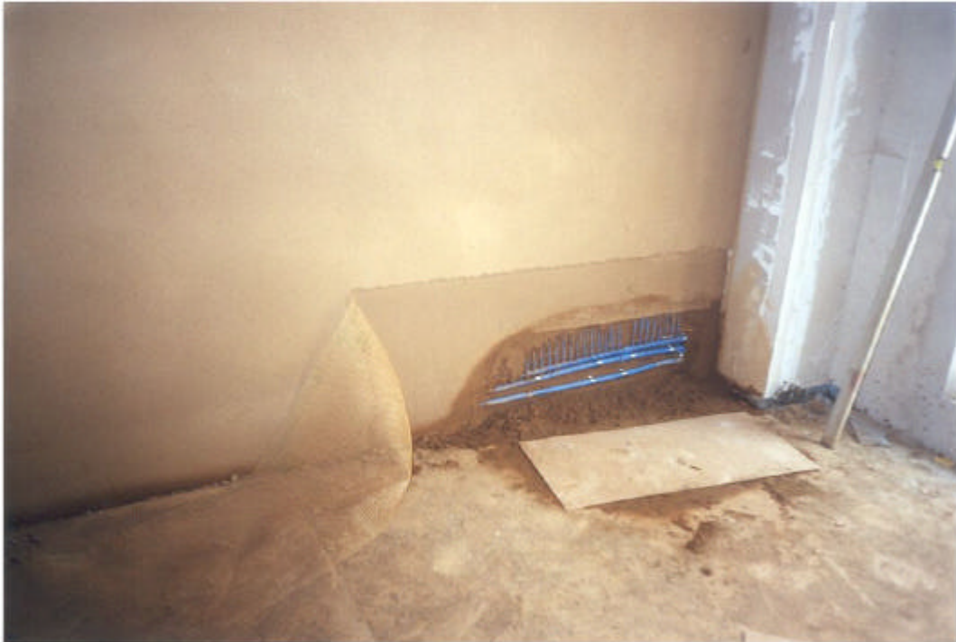
Picture 2: Earthen plaster on a wall-heating-system
