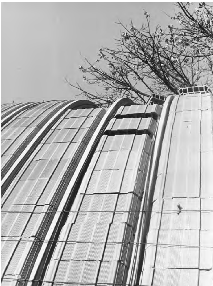
WAITING FOR THE CONCRETE. RODRIGO LEFÈVRE AND NESTOR GOULART REIS FILHO, PERY CAMPOS HOUSE, SÃO PAULO, 1970.
