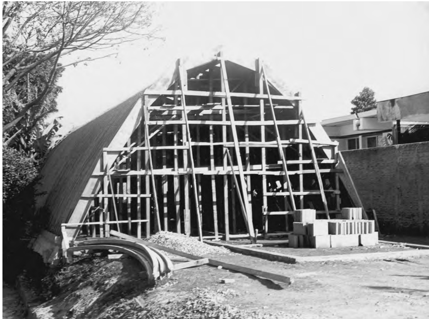
CONSTRUCTION SITE. RODRIGO LEFÈVRE AND NESTOR GOULART REIS FILHO, PERY CAMPOS HOUSE, SÃO PAULO, 1970.
