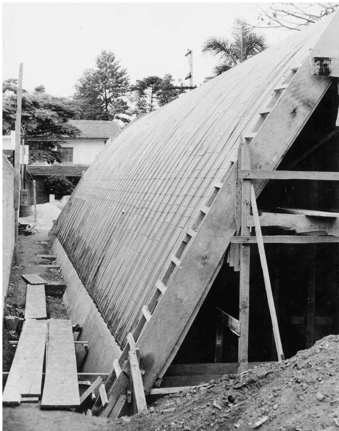
POPULAR CONSTRUCTION TECHNIQUES. RODRIGO LEFÈVRE AND NESTOR GOULART REIS FILHO, PERY CAMPOS HOUSE, SÃO PAULO, 1970.
